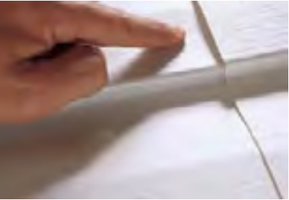
OVER TIME, THE SEAMS ON REGULAR VINYL TEND TO OPEN UP BECAUSE THERE'S NOTHING TO SUPPORT THE SIDING.
